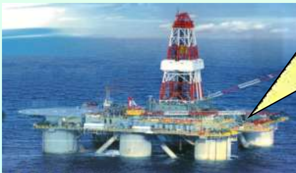
AUTONOMOUS POWER SUPPLY OF MARINE OIL-PRODUCING PLATFORMS
